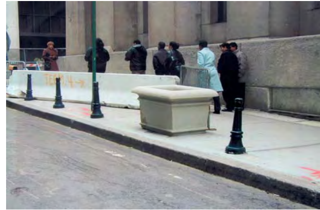
Barrier creates choke point
