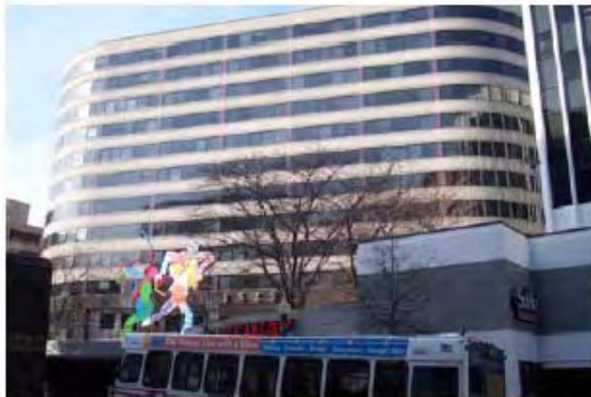
Structure with curtain wall
