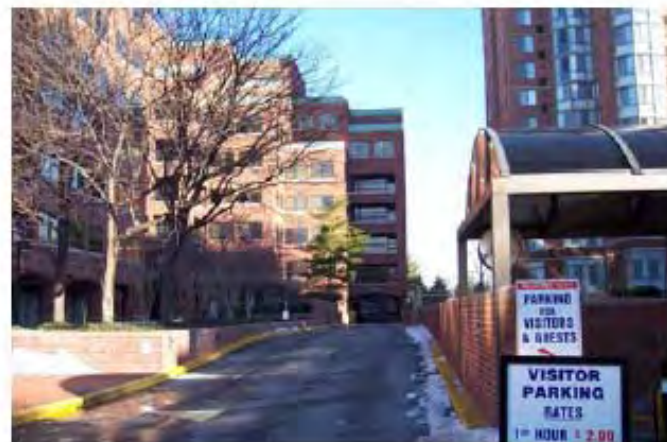
Structure with individual Window
